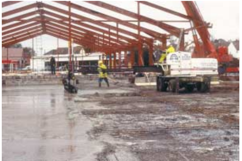
The laser screed being used to lay the external hardstanding.
