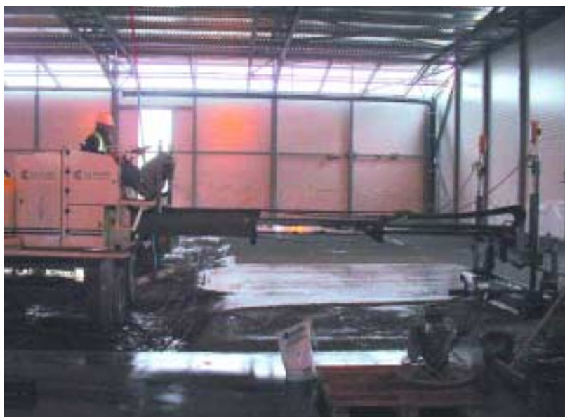
Figure 2: The laser-screed in use on the suspended floor slab.
